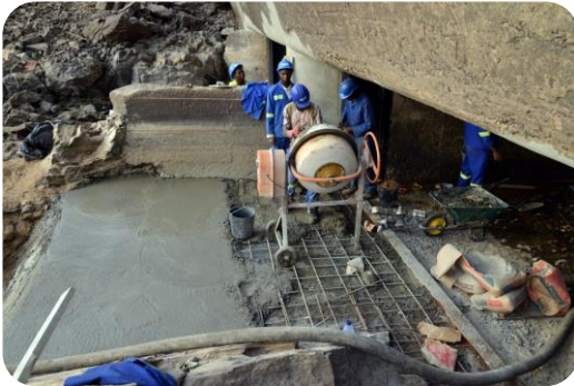
Bottom outlet embedded parts refurbishment on Mavuzi
