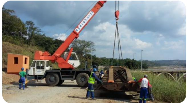
On site gates storage
