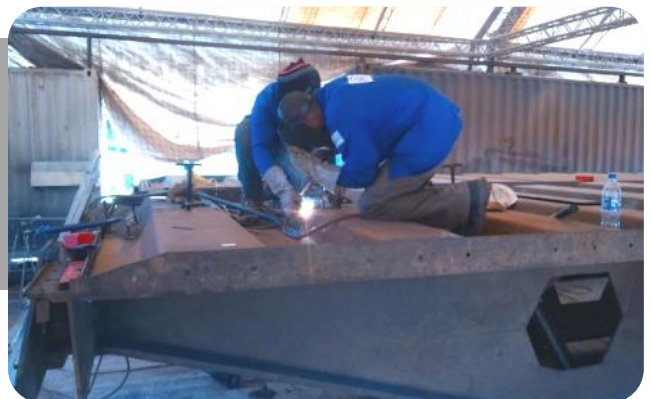
Welding on gate
