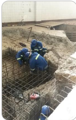
Reinforcement installation
