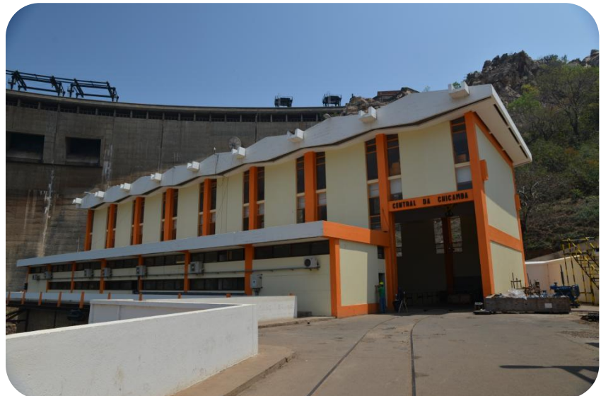
Painting on Chicamba facade
