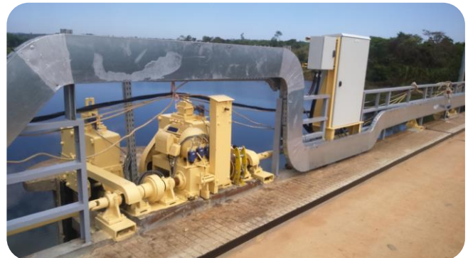
Refurbished motorization and electric box
