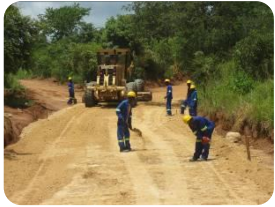
Road sub-layer levelling
