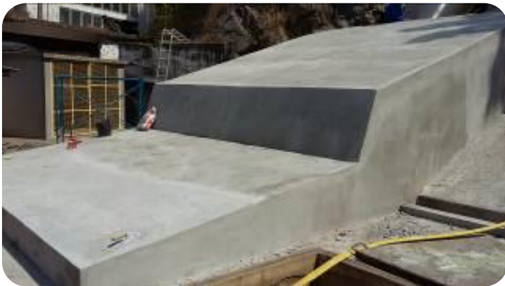
Foundation refurbishment and prestressed wire replacement
