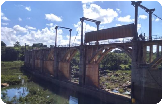
Spillway gates removal with temporary gantry crane
