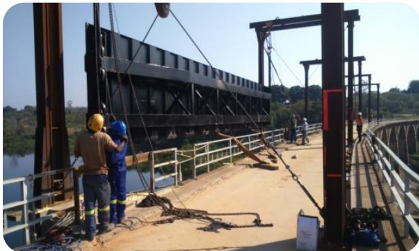
Refurbished gate installation
